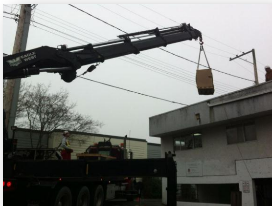
Installation of the new furnace 2012
